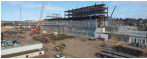
Construction continues on Marquette's new facility
